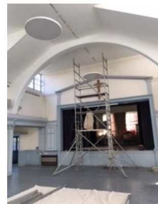
New lighting installed at St Saviour's, April 2023
